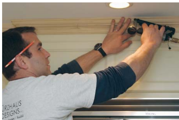
Figure 4. These taller-than-average wall cabinets are sized to leave a balanced reveal on the top rail beneath a crown molding (top left). As long as he's sure he can bring it into the house, the author will build a single cabinet to stand full height under an 11-foot ceiling (top right). Crown molding is normally installed unfinished and painted on site (bottom left).
