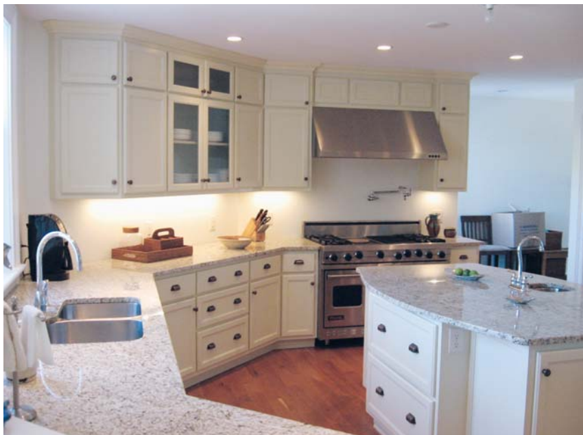
Figure 1. Reveals between drawers and doors are uniformly equal, which gives the cabinetry a distinctive look and a pleasing rhythm. To increase storage space and make access easier, the interiors are left free of unneeded partitions.
