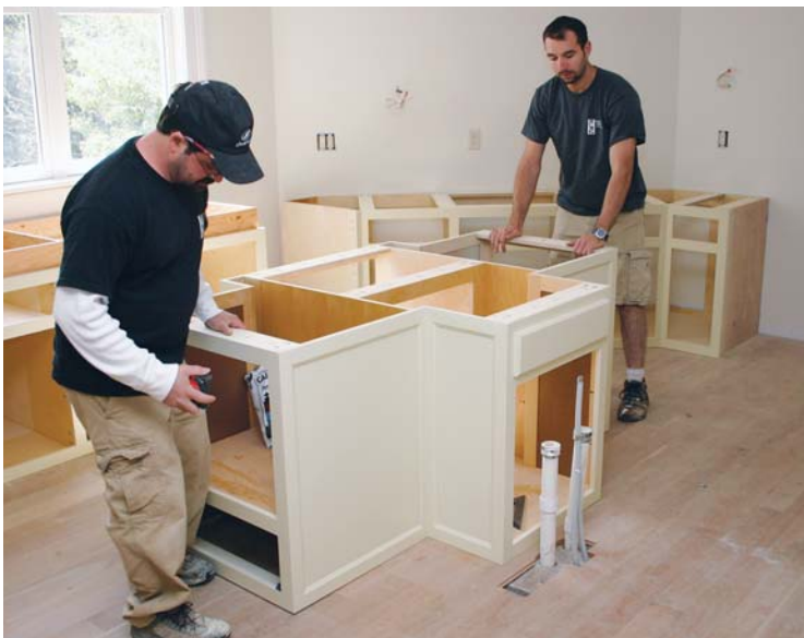
Figure 8. An island cabinet with pilasters and a raised snack bar takes shape (top left). The contiguous face frames are directly connected to a structural, raised-panel back. Interior bracing, partitions, and bottom panels will be pocket-screwed from inside. The author and a helper plot the final position for another island cabinet (bottom left), shown finished in Figure 1. The island above is 9 feet long and weighs more than 1,000 pounds empty. It's supported entirely on four bun feet.
