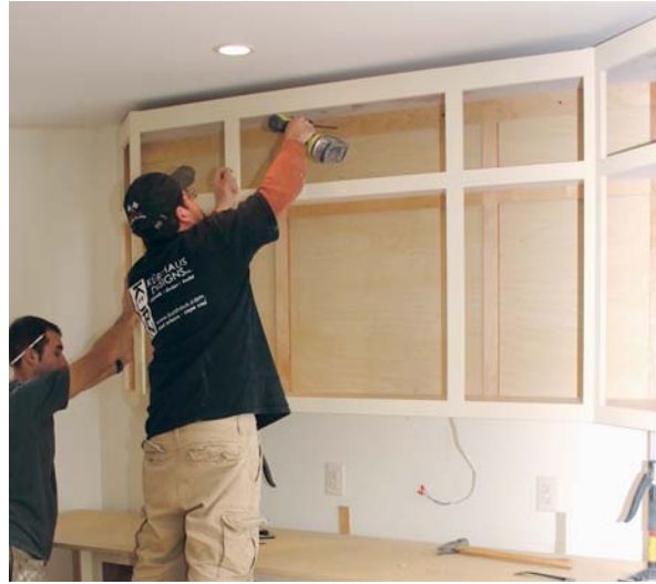
Figure 3. Complete runs of wall and base cabinets are designed and built as single units. The cabinet shown here, seen finished in Figure 1, fills an 8-foot diagonal wall and contains continuous adjustable shelves accessed by a series of doors along its length.
