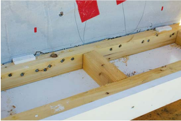
Figure 6. Shims at the back provide a slight slope to the cornice return's cap (above). After the return is finished, the bottom section of the rake soffit can be installed (right).
