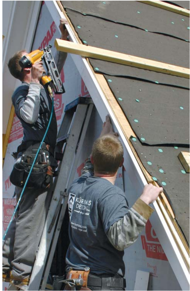
Figure 5. Overhang ladders ripped from 2x8s attach to the gable with TimberLok screws (above left). Since it's mitered at both ends, the carpenters work the PVC trim from the ridge down in sections (above right). Seams are glued with Bond&Fill (left).
