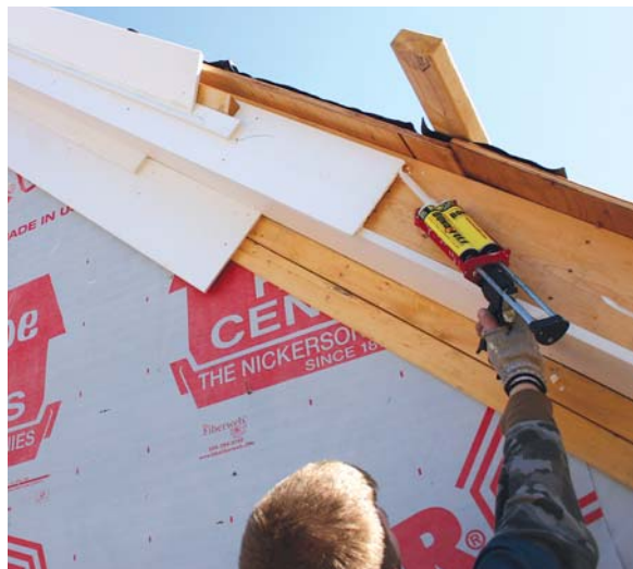
Figure 5. Overhang ladders ripped from 2x8s attach to the gable with TimberLok screws (above left). Since it's mitered at both ends, the carpenters work the PVC trim from the ridge down in sections (above right). Seams are glued with Bond&Fill (left).
